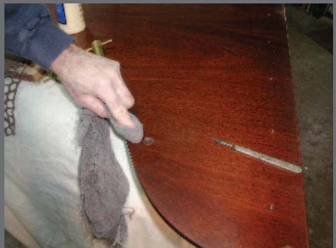
Photo 20 – Clean up the excess glue.
